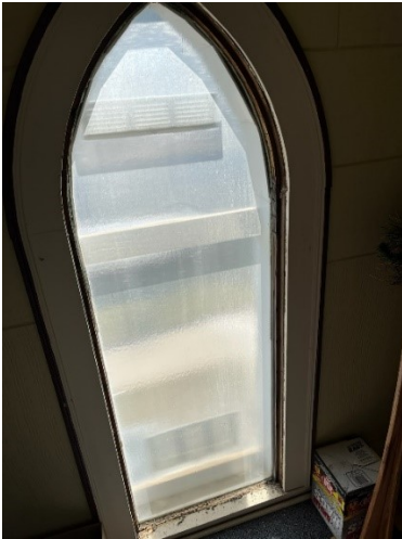
One of the windows with the rolled plate glass. A storm window of old.
