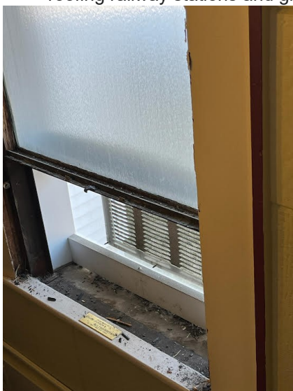
Vent used to let in fresh air before air conditioners. The cloudy glass is rolled glass from the 1800's probably made in New York.
